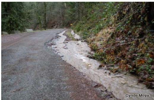
**Figure 1-7.** The result of an undersized/ clogged ditch.
