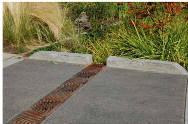
**Figure 1-10.** Decorative trench drain in driveway directs runoff to vegetative landscaping for infiltration.
