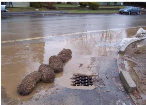
**Figure 1-1.** Improperly placed sediment controls allow polluted stormwater runoff into storm drain which flows directly to surface water.
