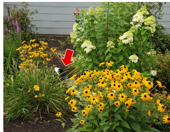
Figure 1-6. A rain garden installed below a downspout.
