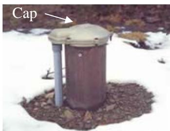
To prevent contaminants from getting down inside the well casing, the driller installs a tight fitting, vermin-proof well cap to prevent easy removal by children or entry of insects or surface water. Well regula-
