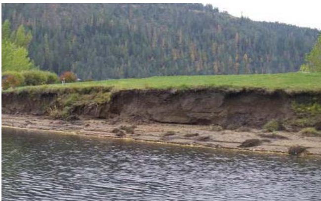
Figure 10-6 Bank erosion caused by boat wakes and flooding. Bank lacks a healthy vegetative buffer.
