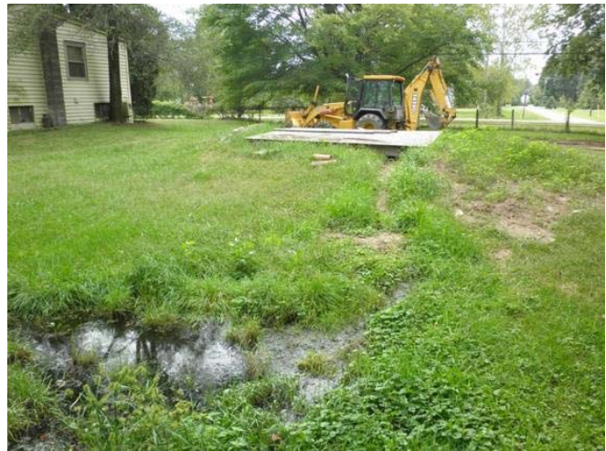
Figure 4-7. Follow the guidelines for a failed system to protect human and environmental health.
