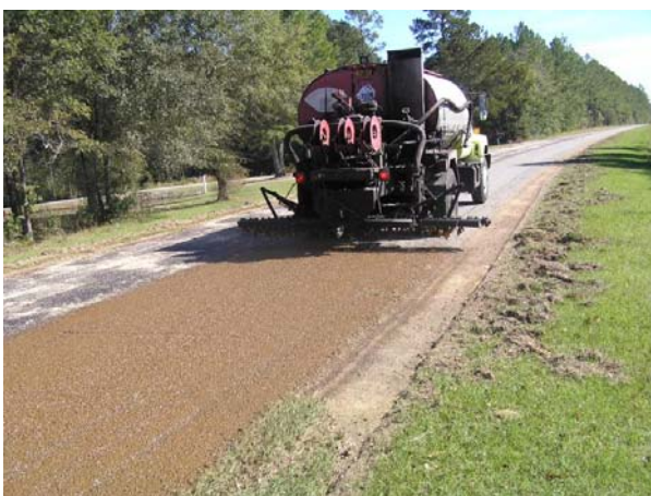
Application of liquid calcium chloride.
