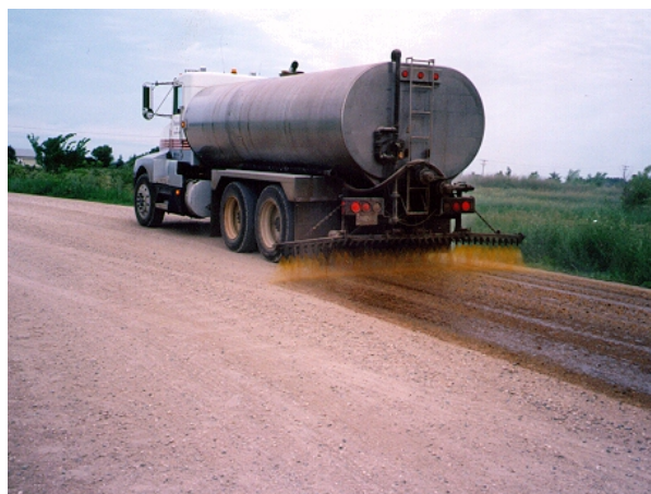
Oil applied to unpaved road.
